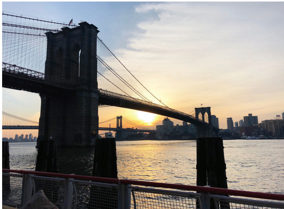
The Brooklyn Bridge in New York.
