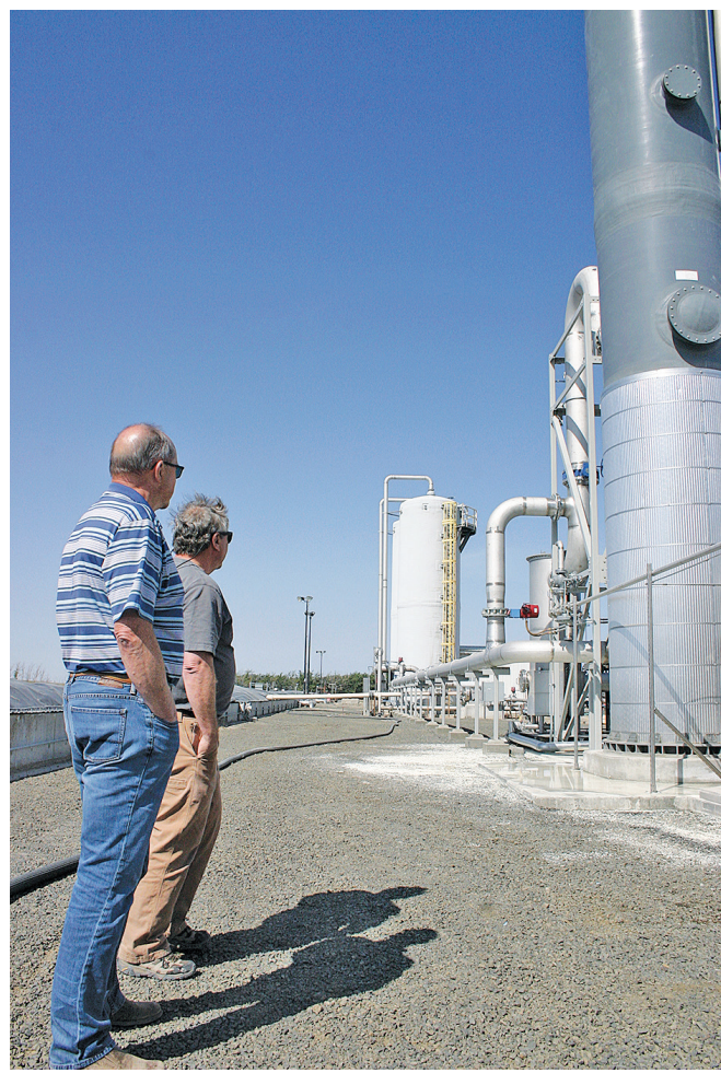
Marty Myers, general manager of Threemile Canyon Farms, and Rick Morck, who helped design and engineer the dairy's manure digester, look at new equipment that converts the gas to 'pipeline quality.' It will be sold to customers in Southern California to make transportation fuel.
