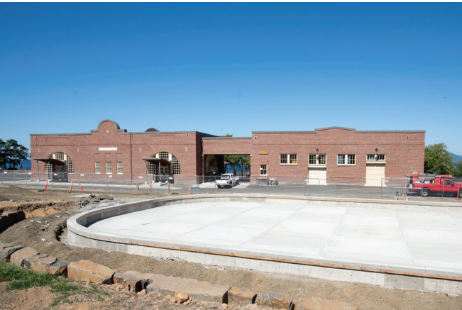
Construction of the pond continues outside the Columbia River Maritime Museum.
