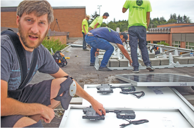
Stephen Shumaker, left, an instructor with Clatsop Community College’s Upward Bound Summer Academy, had his students design a new solar array installed on top of Warrenton High School.
