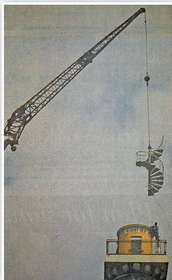
2009 — A crane lowers a section of stairs into place in the Astoria Column. The top of the column was removed so the stairs inside could be replaced.
