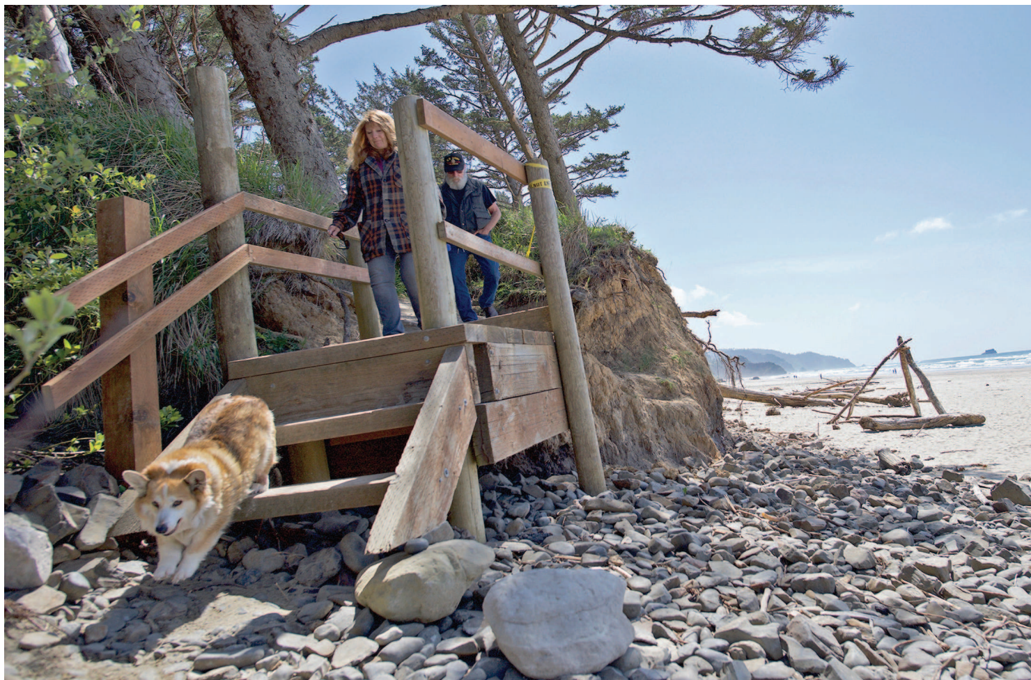
Visitors to Arcadia Beach make their way down damaged stairs.
