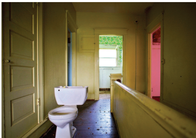
The home does not have working plumbing or electricity and the interior of the house would require extensive renovation.
