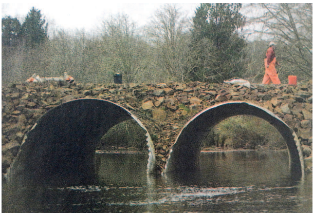
2009 — Gary Johnson, Pacific Northwest National Laboratory research scientist from Battle Ground, Wash., stands atop two large culverts installed in 2004 to restore the diked pasture at Columbia Land Trust’s Kandoll Farm property. The culverts allow for fish passage and the free exchange of water and nutrients between the marsh and the Grays River system.
