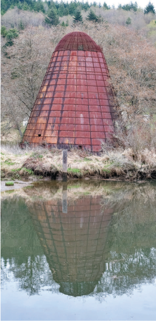
Heavy rust coats the wigwam burner at the former Beaver Lumber Co. sawmill site near Clatskanie.
