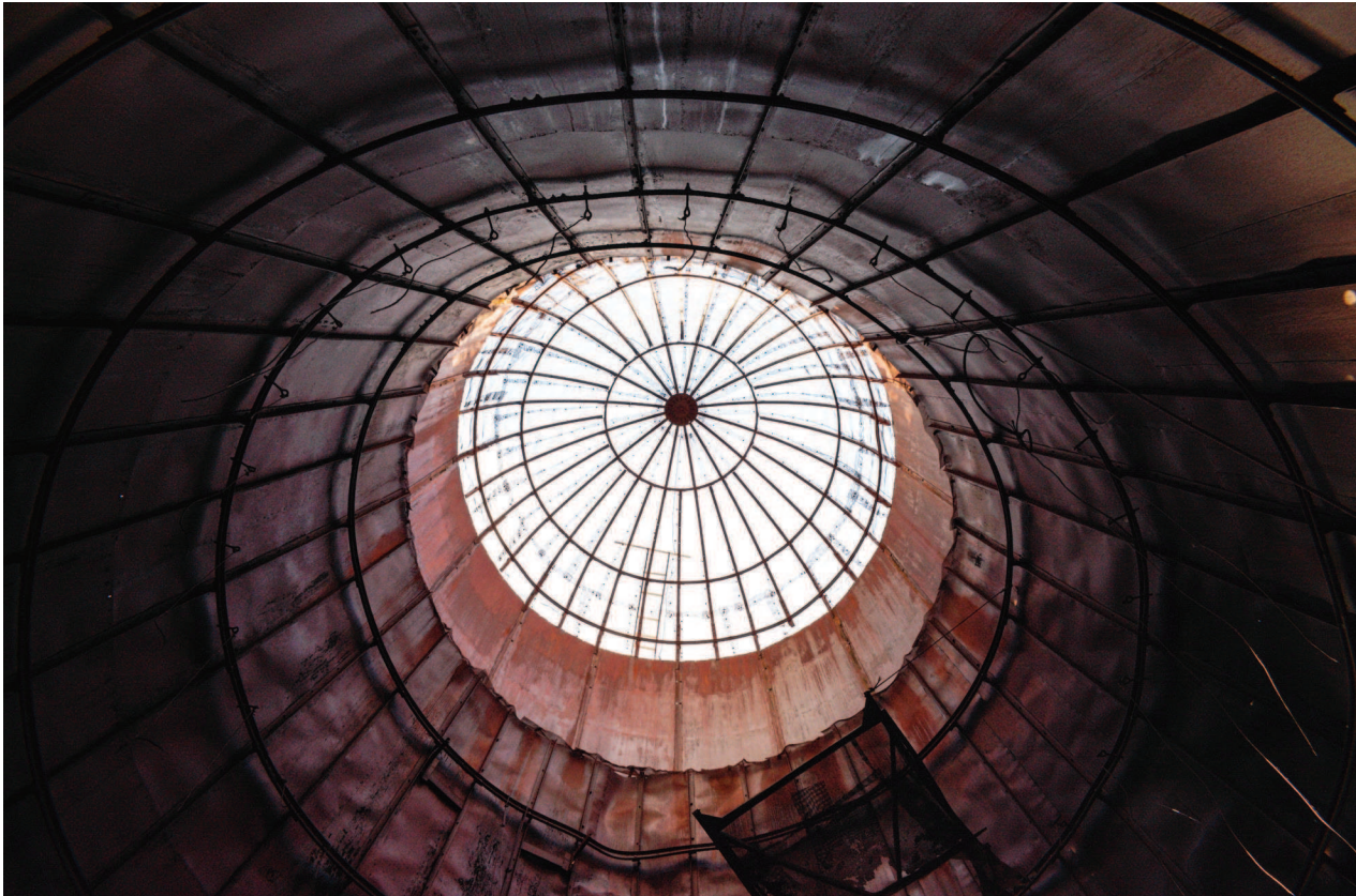
Inside the dome of a retired wigwam waste burner in Hood, Washington.
