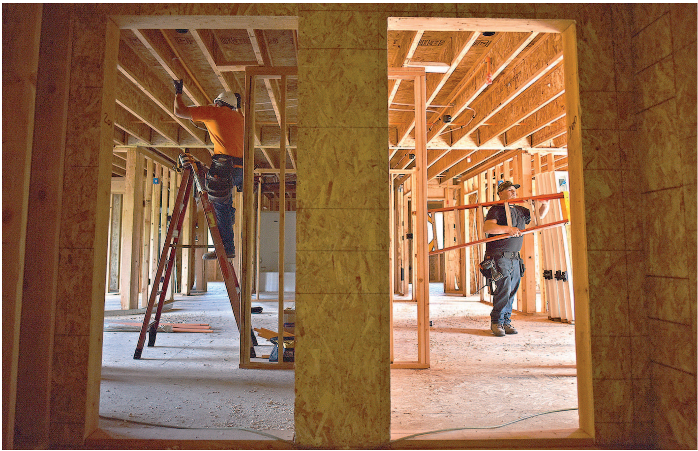
Construction workers build the interior of a housing complex in Warrenton in 2018.
