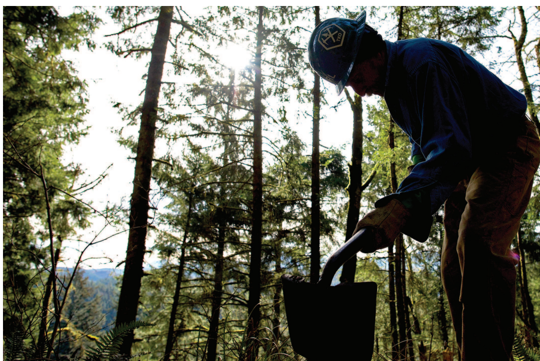
Carl Nyberg works on a trail at Ecola State Park.
