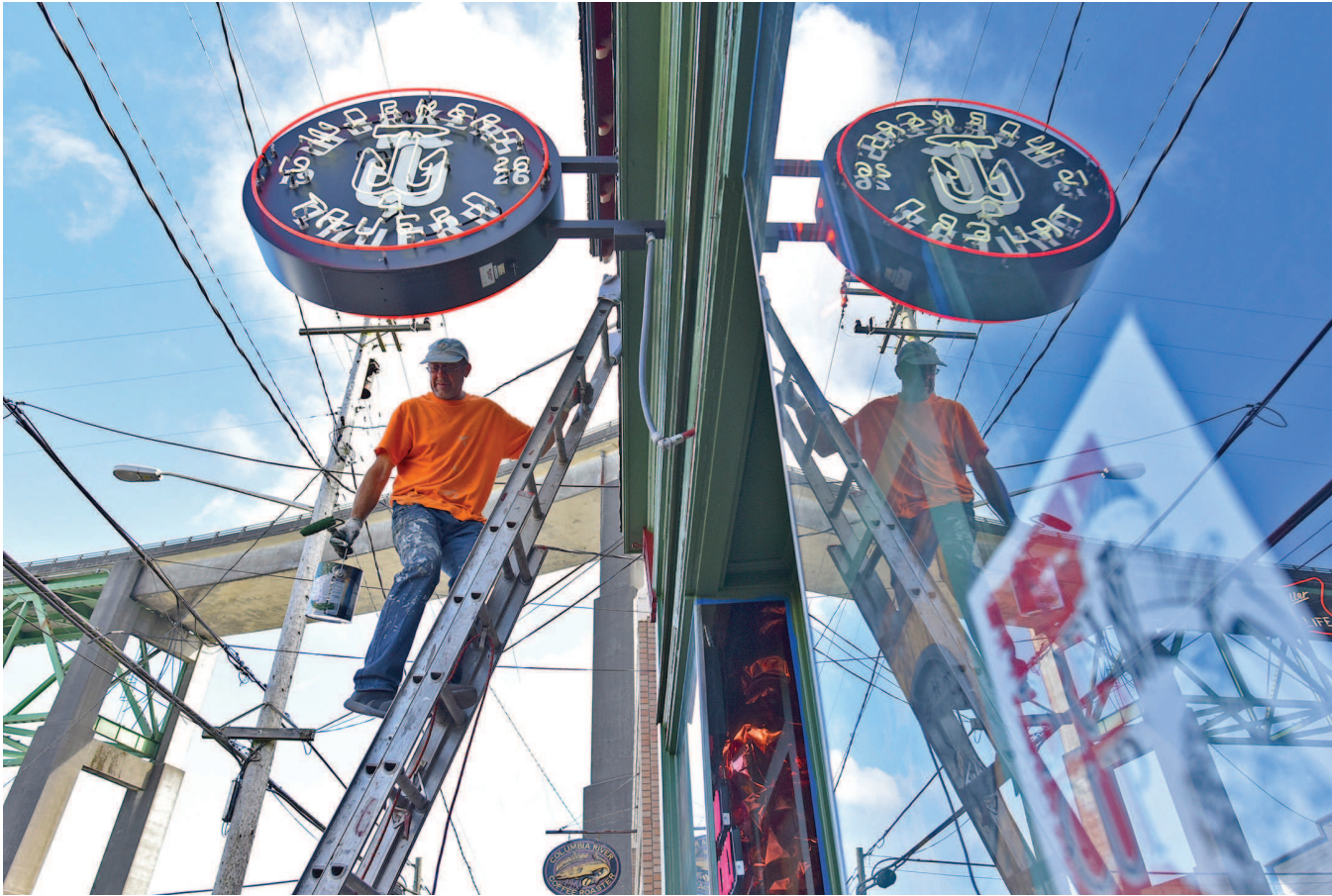
Improvements are made to the facade of Workers Tavern in Uniontown in 2018.
