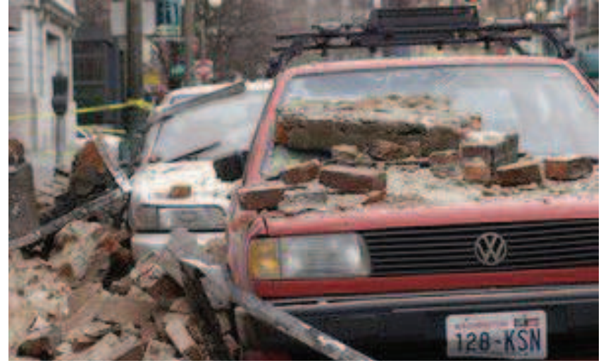
Bricks that fell from an earthquake cover parked cars in Seattle's Pioneer Square district in 2001.
