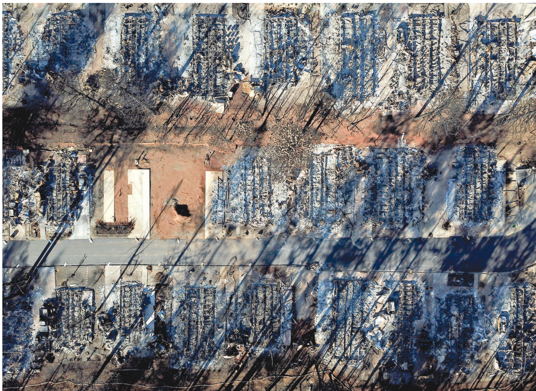
Nearly every structure in this mobile home park in Paradise, California, was destroyed in the Camp Fire.
