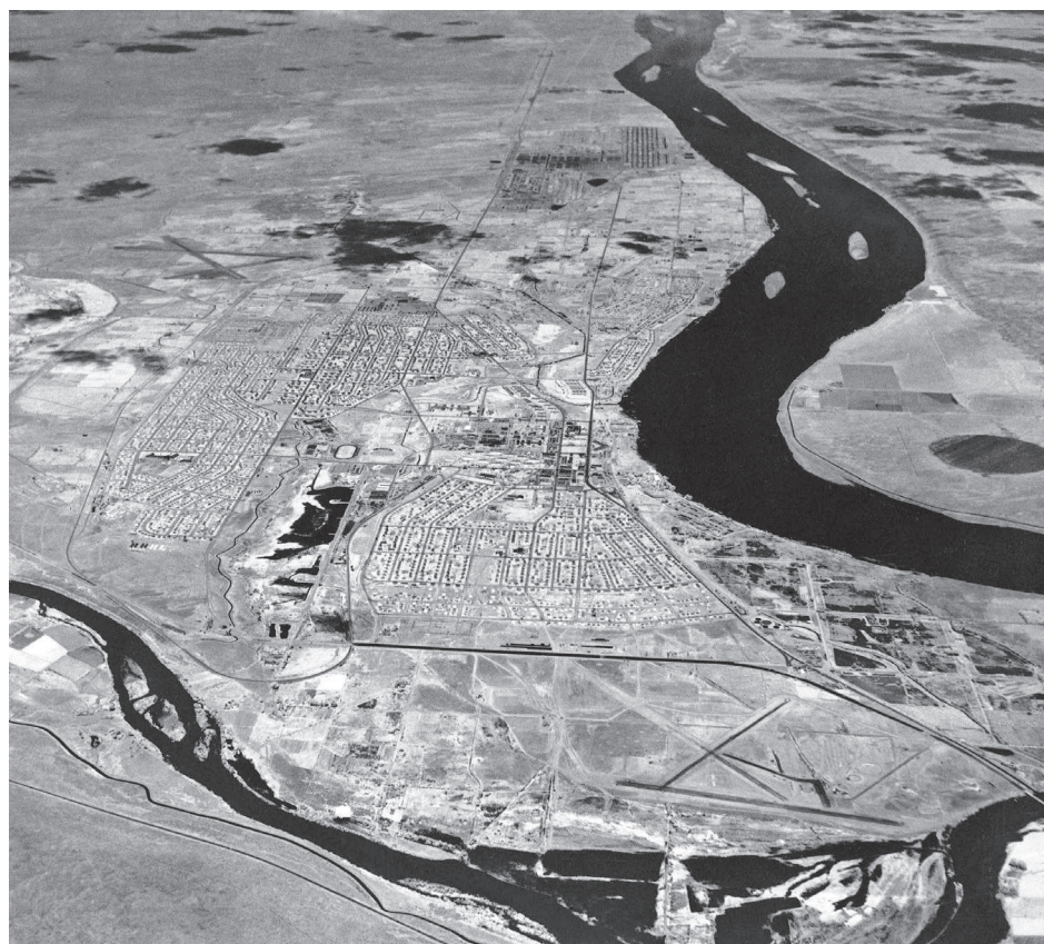
An undated aerial view of part of the Hanford nuclear reservation.
