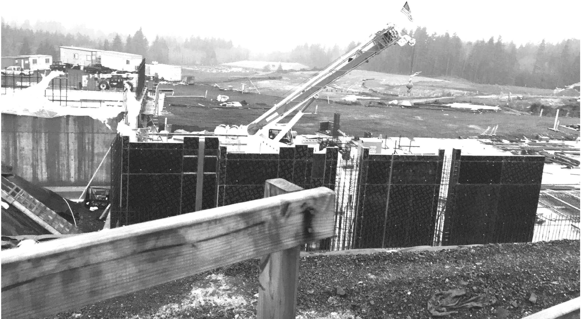
Crane lifts rebar and other material onto the site.
