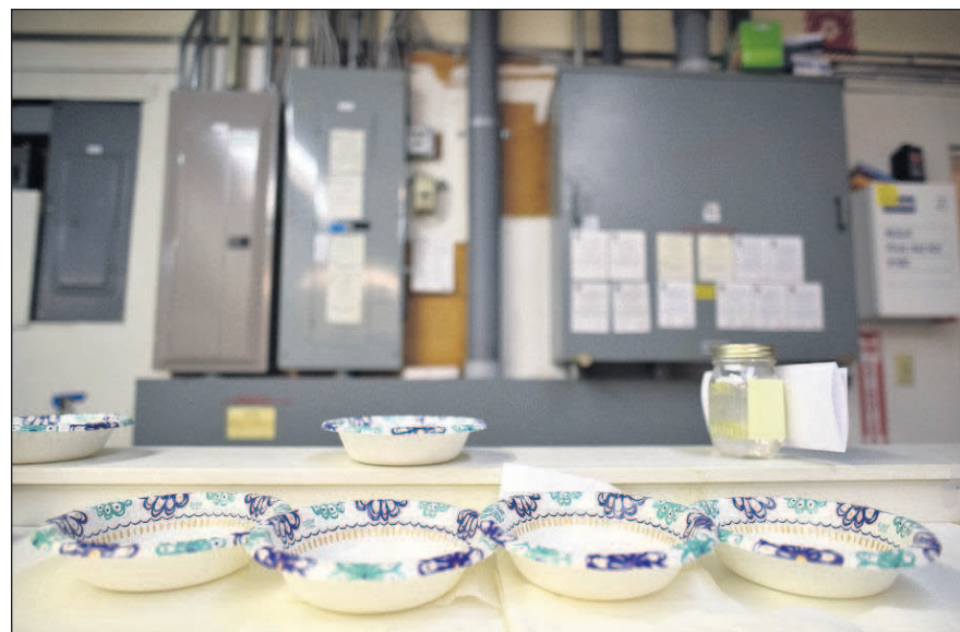
Bowls are set up at Cannon Beach City Hall to collect water dripping from the ceiling.
