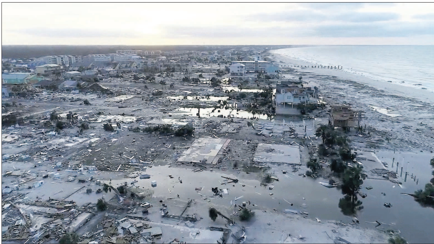
In this image from video, damage from Hurricane Michael is seen in Mexico Beach, Fla.
