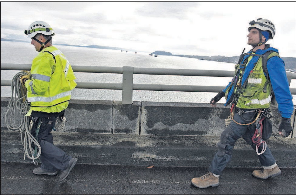
Dale Poorman, left, and Benjamin Barkan walk along the Astoria Bridge before performing an inspection.
