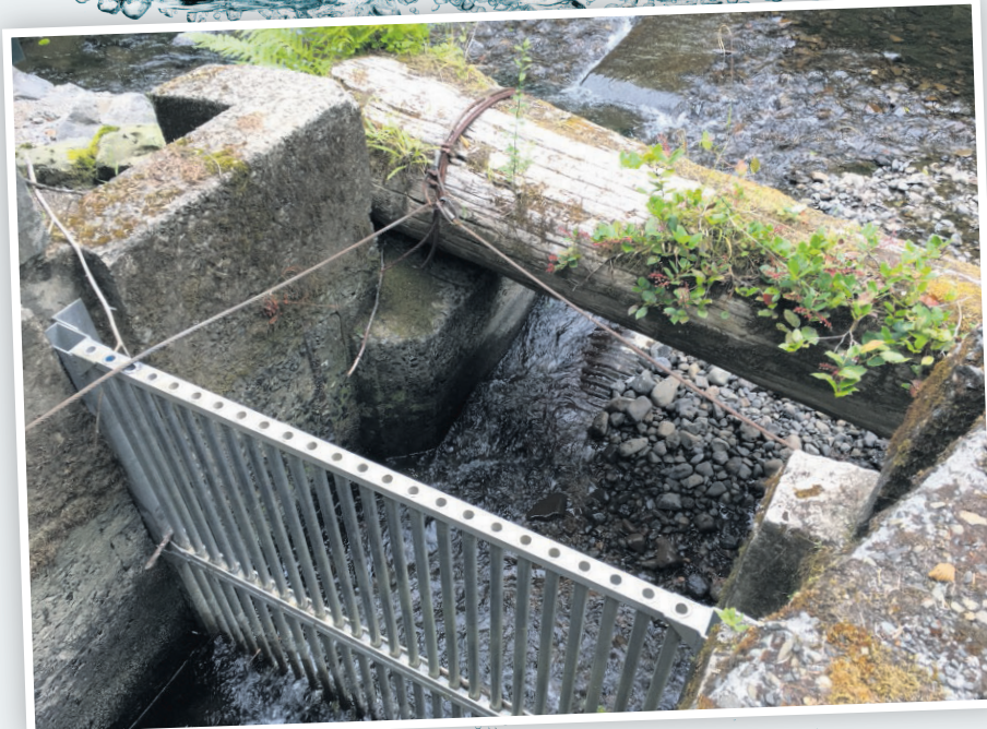
Fish diversion at the system's headwaters.
