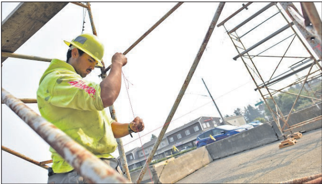
Ollie Baker makes adjustments to a temporary bridge spanning U.S. Highway 101 in Seaside for Hood to Coast runners.
