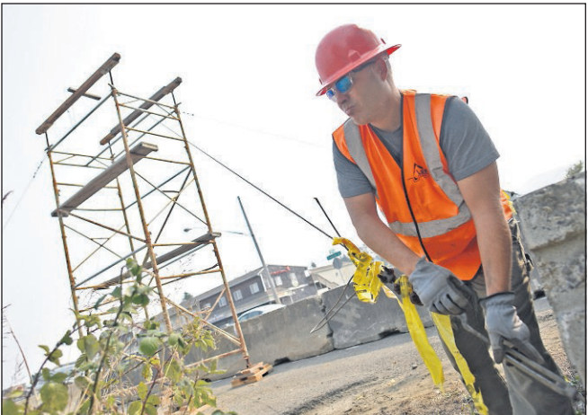
Dennis Thomas works on the temporary bridge across U.S. Highway 101 for runners participating in Hood to Coast in Seaside.
