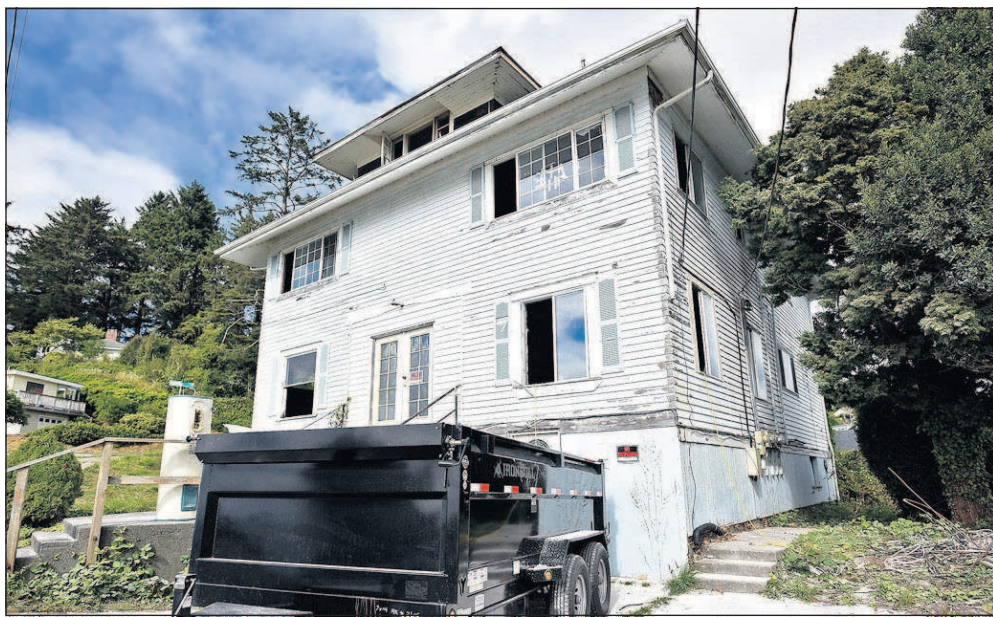
A house near Uniontown in Astoria is under renovation.
