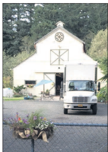
The owner of the Neacoxie Creek Barn was fined for its use as a party venue without a certificate of occupancy.
