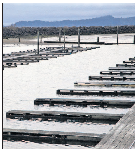
Parts of the Port of Chinook mooring basin are inaccessible at low tide due to silt buildup.
