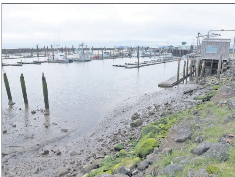
Silt continues to plague the Port of Chinook.
