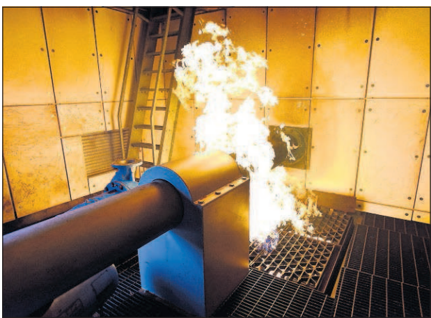
Several of the rooms in the facility are designed to mimic conditions found on ships.
