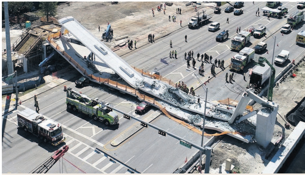
The collapsed pedestrian bridge at Florida International University.
