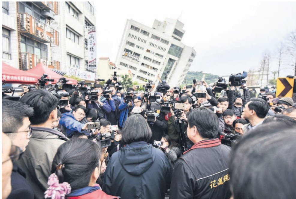
Taiwan Presidential Office President Tsai Ing-wen, center back-facing, is briefed today at the site of a collapsed building from an earthquake in Hualien, southeastern Taiwan.
