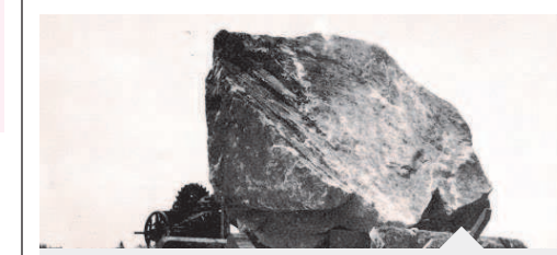
CHINOOK OBSERVER ARCHIVES Giant boulders like this were used to build the Columbia River jetties.
