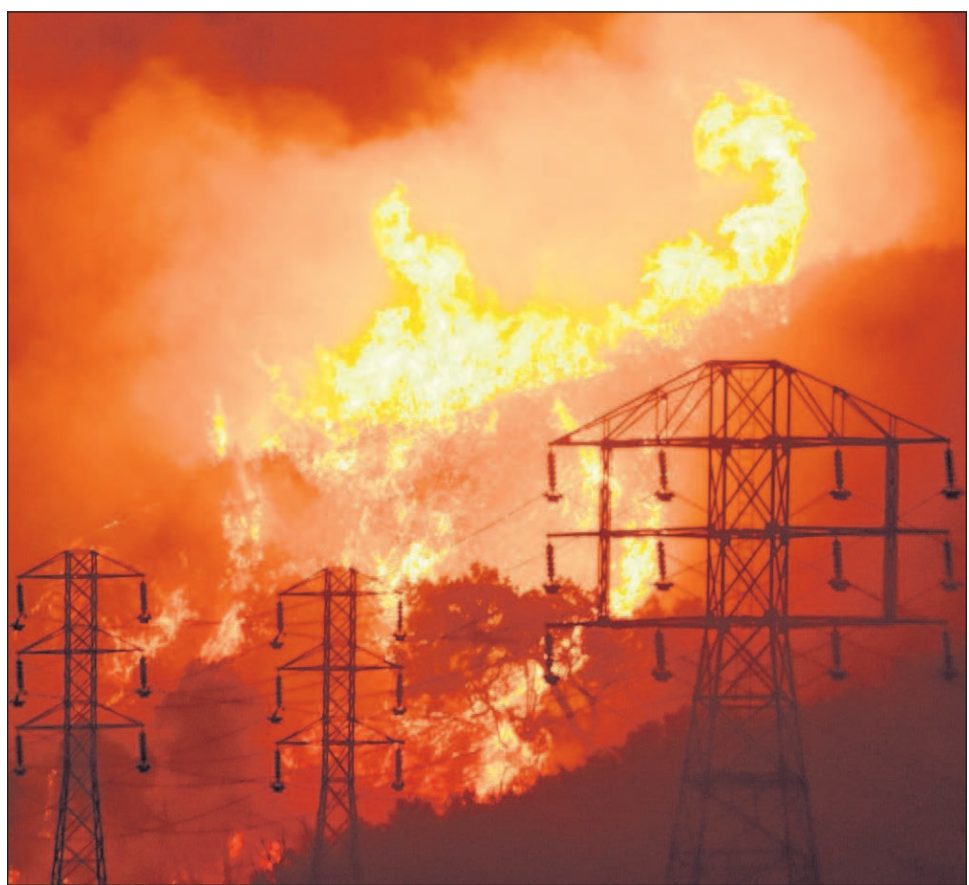
Santa Barbara County Fire Department
