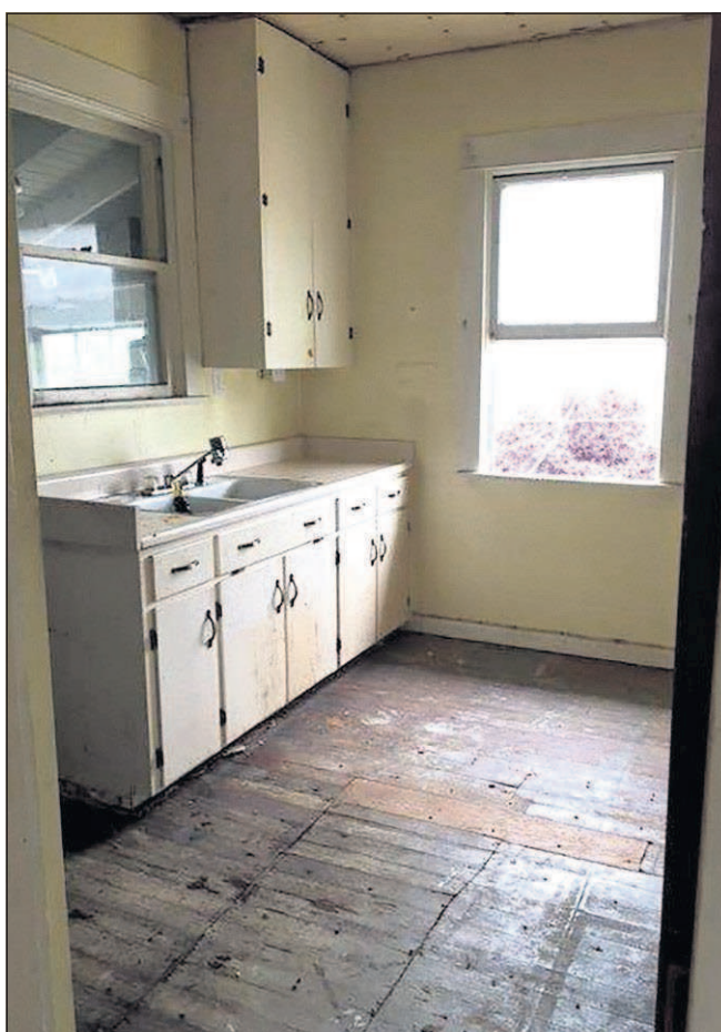
After removing nearly 100,000 pounds of debris from this Alderbrook home, the property was restored and will now be put on the market.
