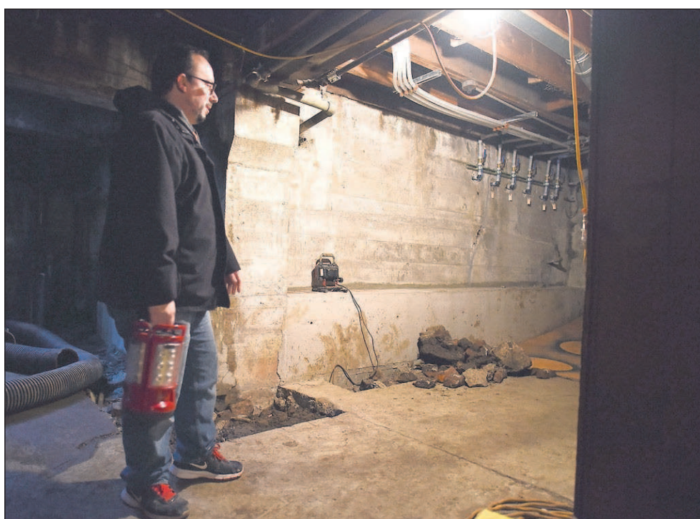
Marcus Liotta looks over work done to improve the foundation.
