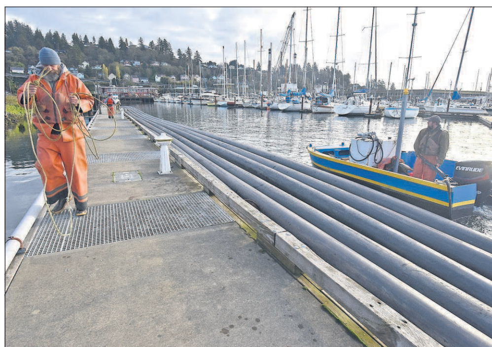
Workers prepare pipe Monday to be moved into place for a dredging operation at the West End Mooring Basin at the Port of Astoria.
