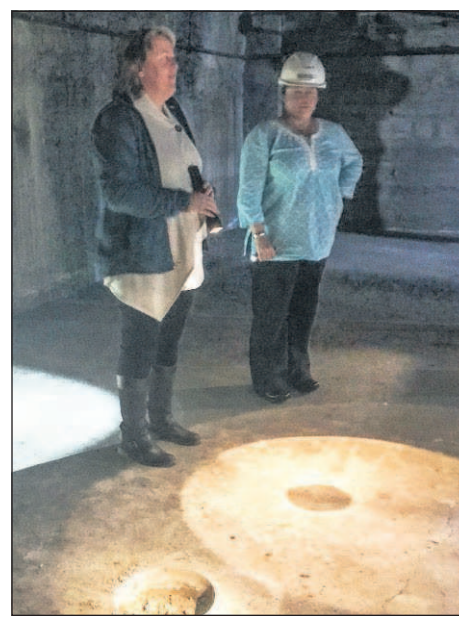
Julie Garver, left, the housing development director for Innovative Housing Inc., points out a boring the group did to test soils.
