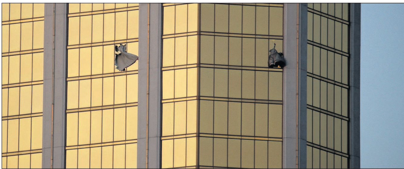
Drapes billow out of broken windows at the Mandalay Bay resort and casino Monday on the Las Vegas Strip following a deadly shooting at a music festival in Las Vegas. A gunman was found dead inside a hotel room.
