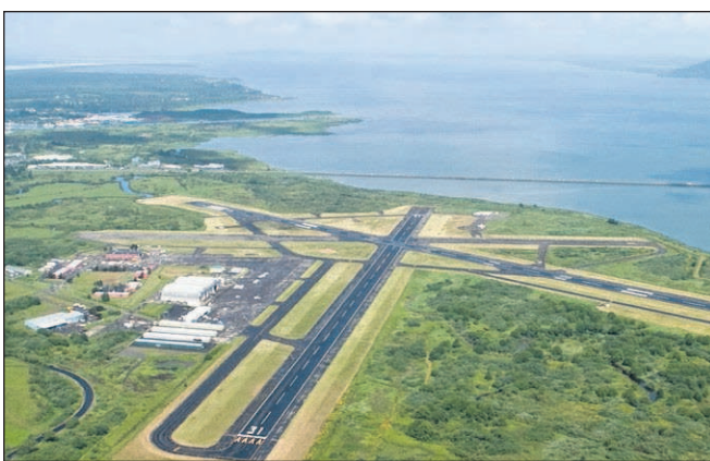
Corpac Construction was hired by the Port last year to rehab runway 13-31, in the foreground.
