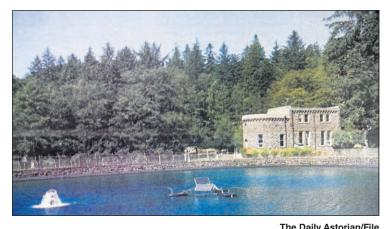
Reservoir 2, adjacent to Shively Park, holds 6 million gallons of water and serves most of the city below the elevation 190 feet. The reservoir, built of brick in 1895, must be covered to meet federal drinking water rules.
