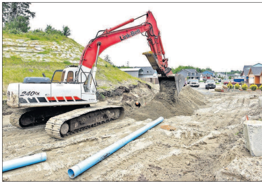
Construction work continues at one of Warrenton’s new housing developments.
