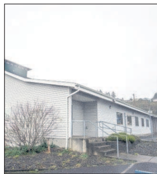
Joshua Bessex/The Daily Astorian Shooting Stars Child Development Center wants to move into the former Oregon State Police station near the Port of Astoria.
