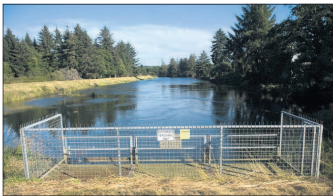
The Skipanon Water Control District has asserted jurisdiction over the Eighth Street Dam.
