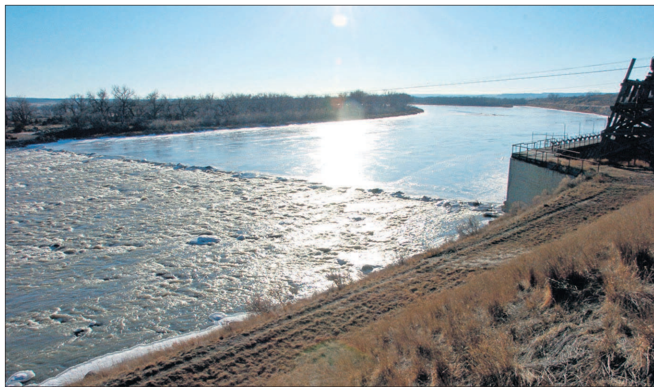
The Yellowstone River flows over the Intake Diversion Dam, a rock structure that captures water for agriculture, northeast of Glendive, Mont., near the North Dakota border.
