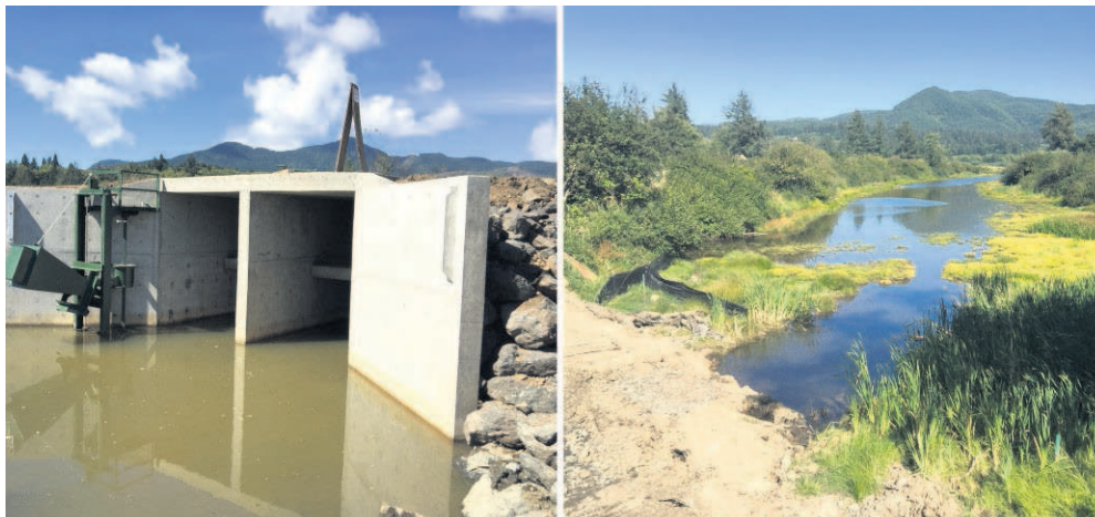
The McDonald Slough Reconnection Project, completed in September, replaced a failing and undersized tide gate with a fish friendly structure, improving habitat access and water quality.
