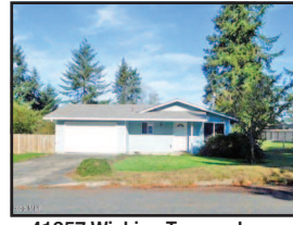
41957 Wickiup Terrace Lane $239,000
