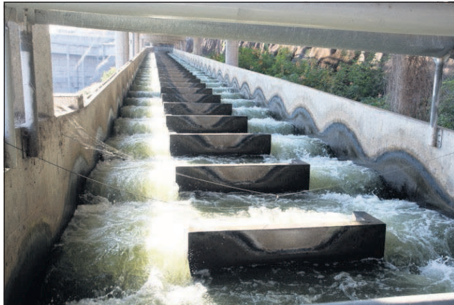
Photos by Dean Hare/The Moscow-Pullman Daily News ABOVE: Water flows through a fish ladder at Lower Granite Dam on the Snake River in Washington state. RIGHT: Matt Corsi, right, and Brian Knoth, left, both fisheries biologists with the Idaho Department of Fish and Game, examine a steelhead lifted from the data recording tank at the Lower Granite Dam fish facility on the Snake River in Washington state.
