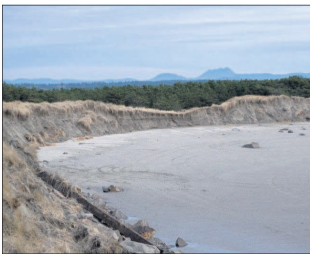
State Department of Geology and Mineral Industries By 2013, the foredune at the root of the South Jetty was in danger of breaching, allowing water past the jetty and directly into Trestle Bay. Such a breach could change the hydrology around the multibillion-dollar Columbia River shipping channel.
