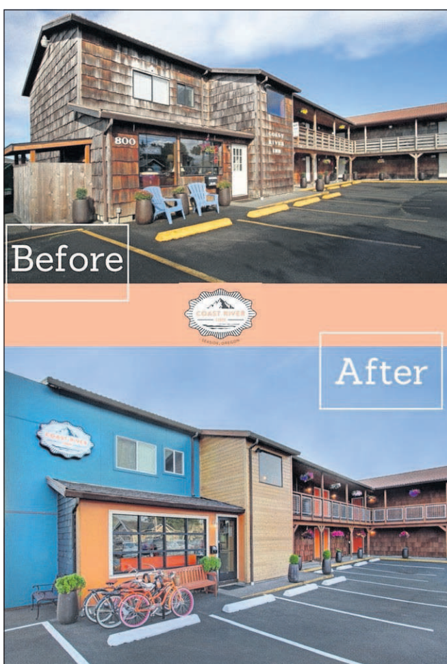
This image from Seaside Lodging compares the Coast River Inn before its renovation, started last fall, and after.
