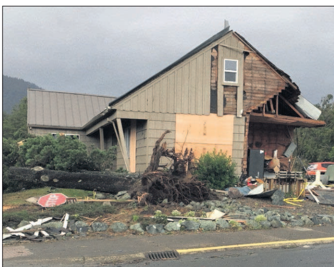
R.J. Marx/The Daily Astorian Damage along Laneda Avenue on Sunday.
