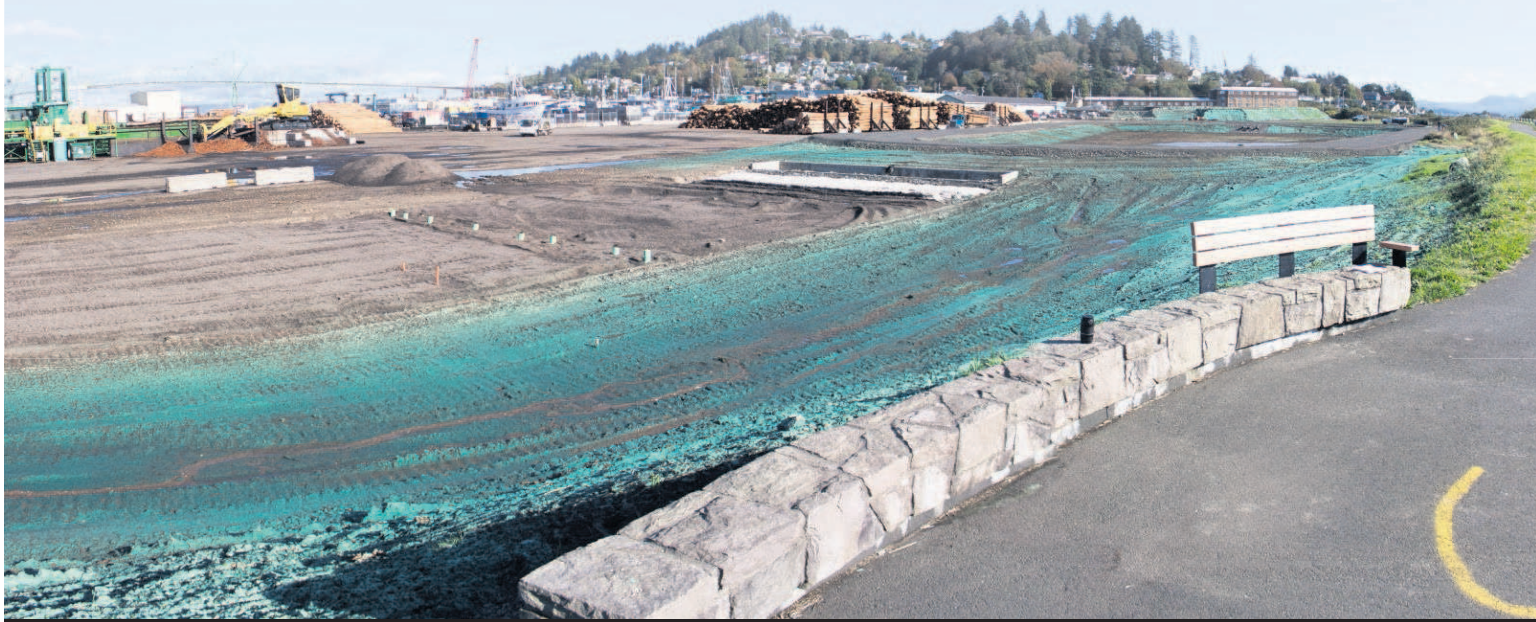
BELOW: The public has a full view of the Port of Astoria's more than 2-acre stormwater treatment system on the western edge of Pier 3. The Port will also build an educational kiosk explaining how the system of settling ponds and bioswales works. Edward Stratton/The Daily Astorian
