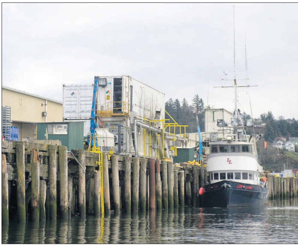
The Port of Astoria has received $1.54 million from the state Department of Transportation's ConnectOregon infrastructure grant program. The money will be used as a local match for funding from Federal Emergency Management Agency to repair storm damage on Pier 2, seen above, and throughout the central waterfront.
