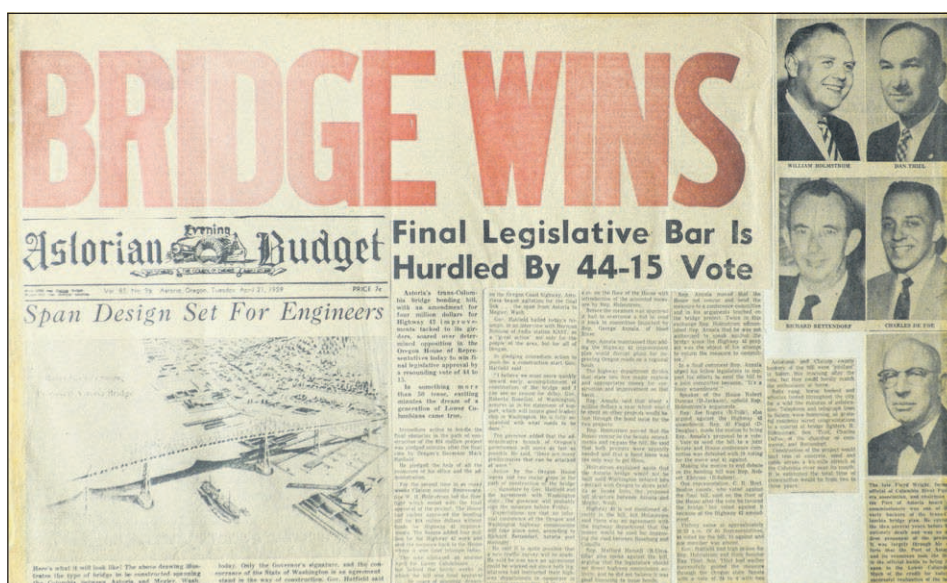
The Astoria Bridge project is announced April 21, 1959, after clearing its final legislative hurdle by a 44-15 vote in the Oregon Legislature.
